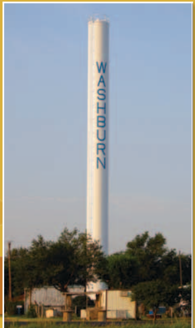
The community of Washburn, located in Armstrong County, received Community Development Block Grant funding for a new standpipe water tank.
